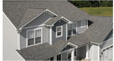
ROOFING AND VENTILATION
