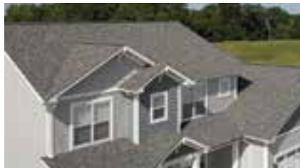
ROOFING AND VENTILATION
