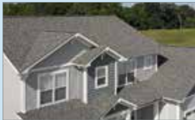
Roofing and Ventilation
